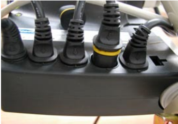
Connected the motor to the control unit.
