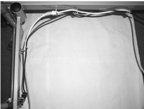
Wiring of the bed end motor (head).
