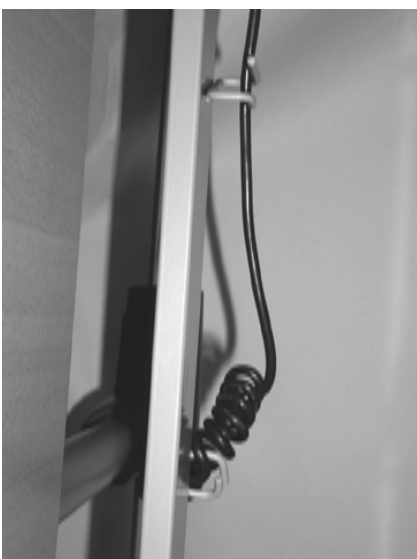
Wiring at the lifting motor, head end.
