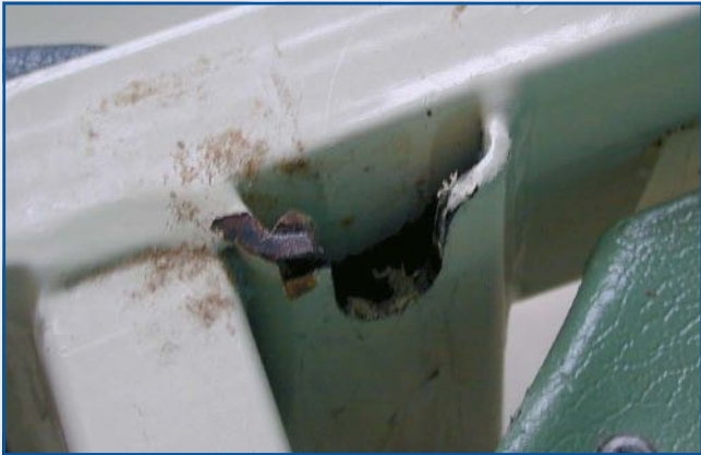
Worn or damaged bed frames
